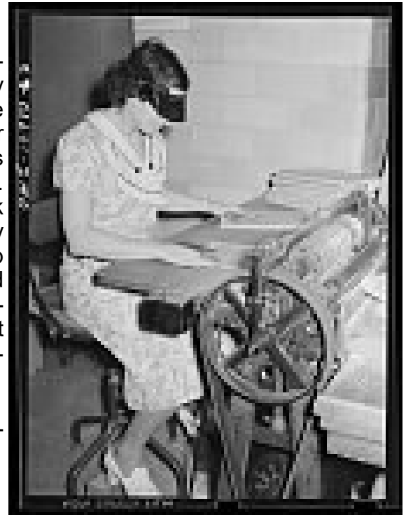
Title: Washington, D.C. Flatbed, single-way postage stamp perforating machine at the United States Bureau of Engraving and Printing From the Library of Congress Created/Published 1938 Arthur Rothstein, photographer
